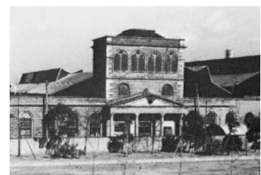
Fig.12. Main Building of Ordnance Factory (1873)
